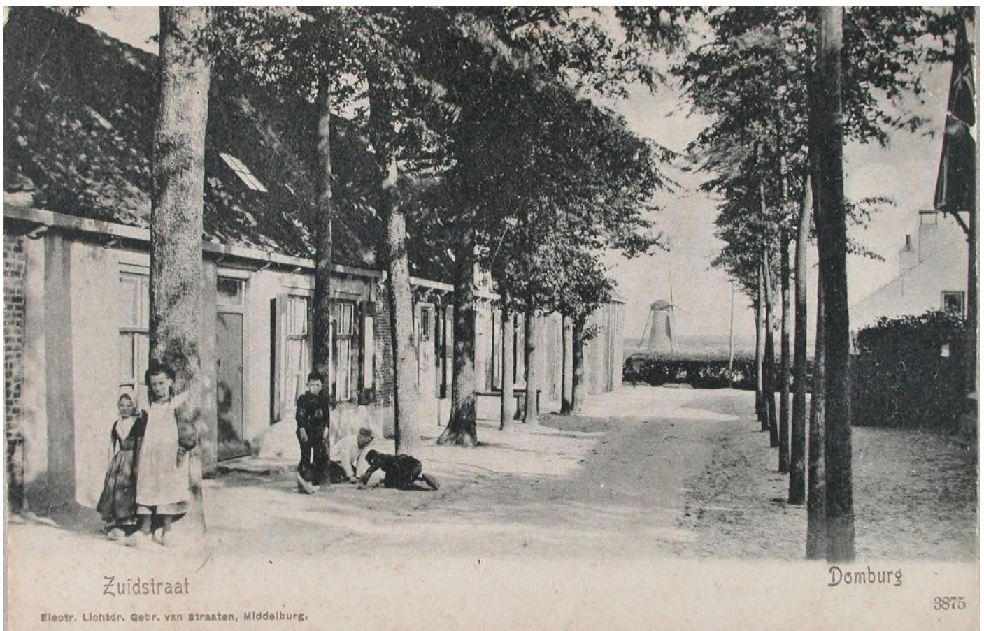
Fig. 14 Picture postcard with Zuidstraat seen from the north by publisher Gebr. Van Straaten. In the back on the right is the "small house" at the research site. Source: Beeldbank Zeeuwse Bibliotheek, recordnr. 4496.
